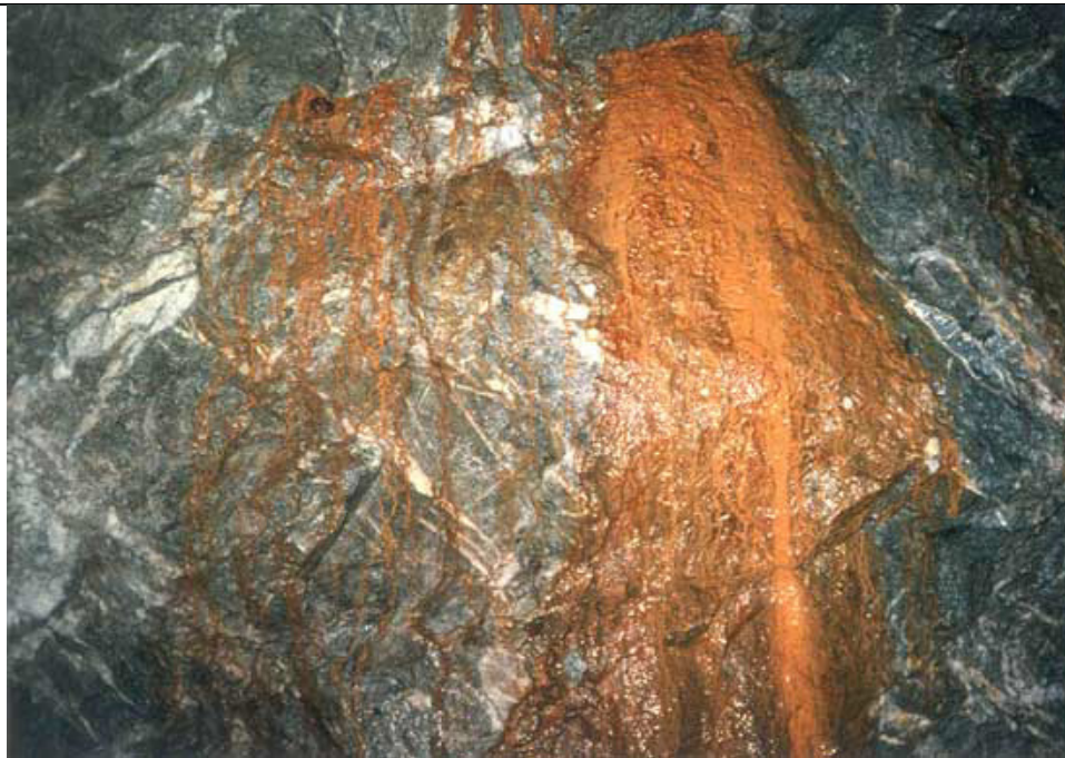
Figure 1: Acid drainage is red or orange because of the iron in it. Acid on tunnel walls at Kensington gold mine (Southeast Alaska). Photo - D. Chambers.
